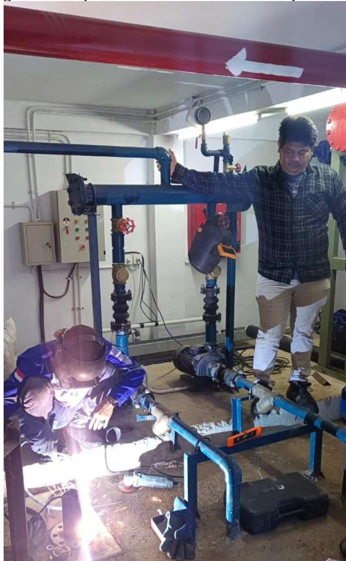
Gambar 1. Proses Pengelasan Pipa Hydrant
